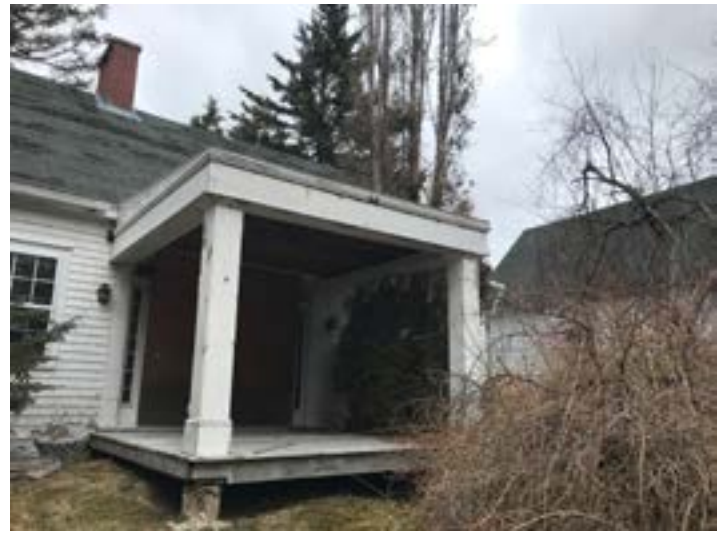
13. The porch on the east side of the building
